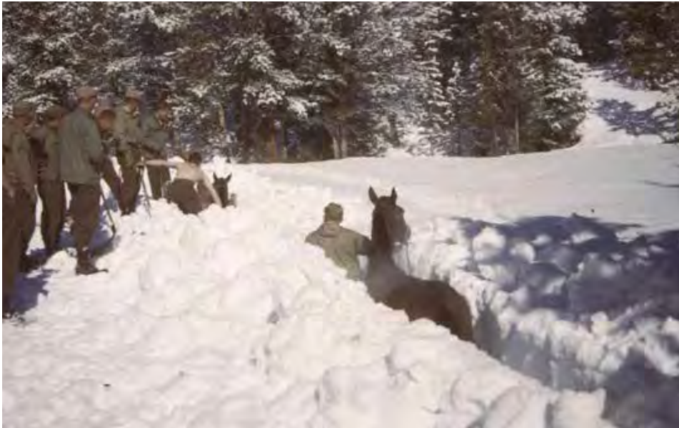
Mule trenches Camp Hale, DPL TMD-703
