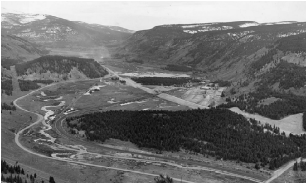
Camp Hale during construction, 1942, DPL: TMD-588
