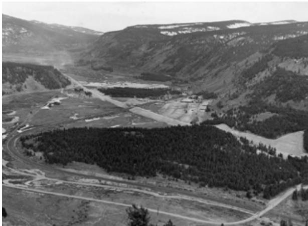
Camp Hale during construction, 1942, DPL: TMD-588
