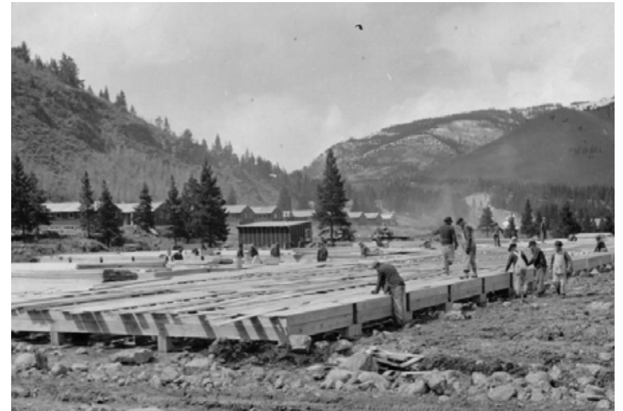
Camp Hale during construction, 1942, DPL: TMD-590
